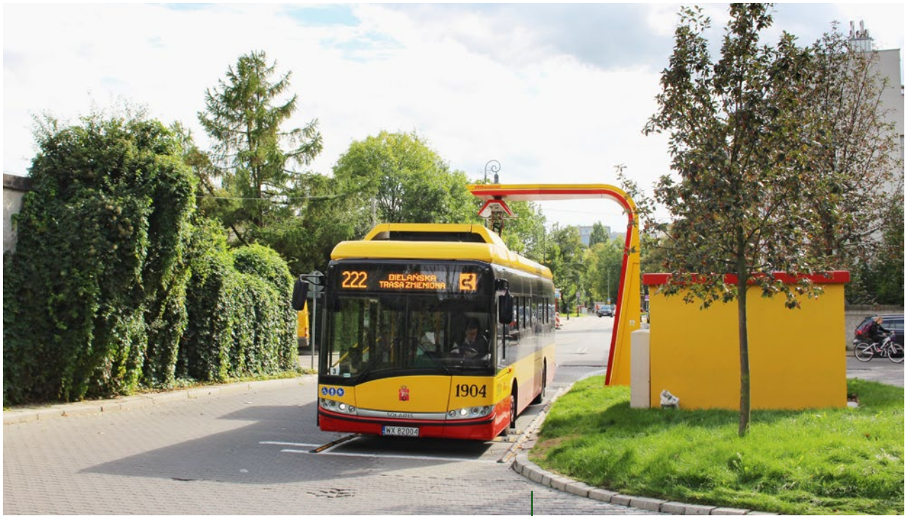
Street charging station on the Spartańska terminus
