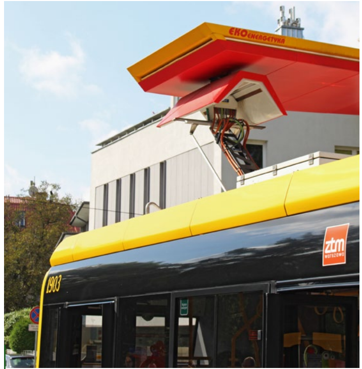
Pantograph charging of a Solaris bus
